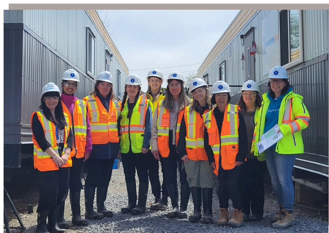
Photo of Grandview Kids Therapy Working Group touring the construction site.
